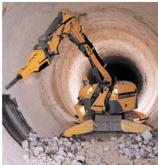
TYPICAL KILN TEAR-OUT USING A BROKK (FIG 2)
