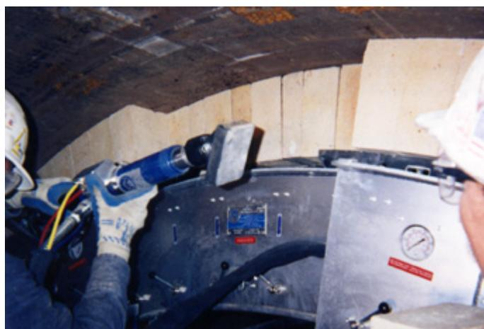
**TYPICAL SETTING OF THE FINGER-TIP CONTROLLED JACK PRIOR TO MOVING THE ARCH AND KEYING THE COURSE (FIG 10)**
