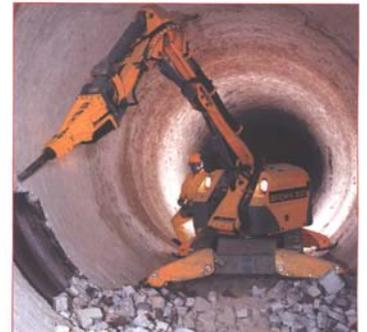
Figure 2. Typical kiln tear-out using a Brokk.
