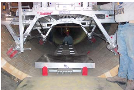
Brake system to hold carts anywhere on trac
